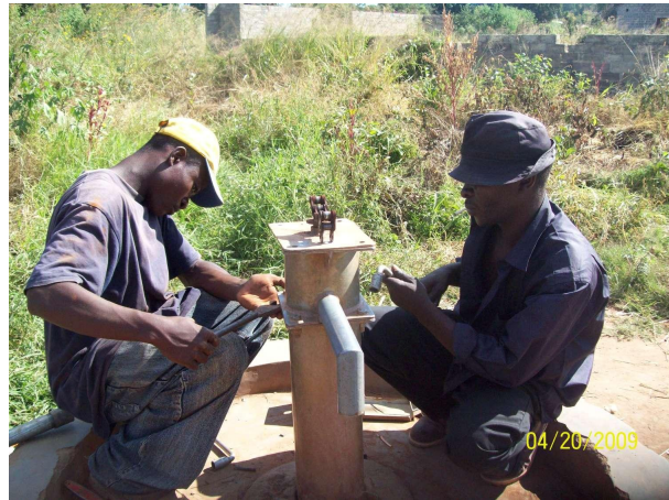
Still working on the pump
