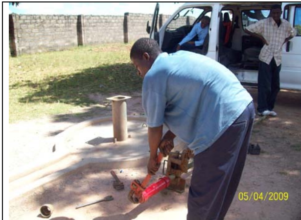
Kapuka Mubanga one of PR crew fitting the new cylinder
