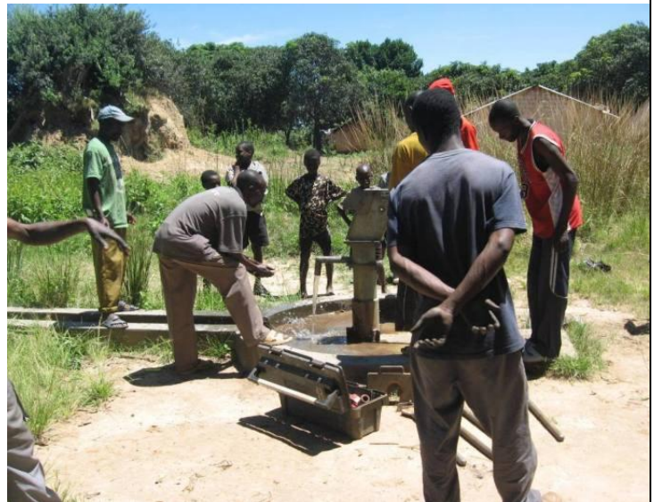
The repairs are completed and clean water is available to the community.
