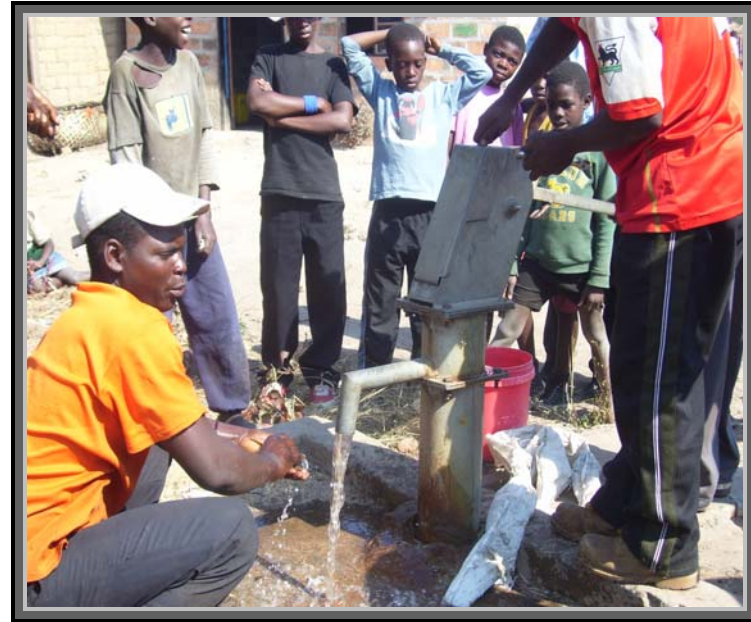
Final touches, but we have water running though.
