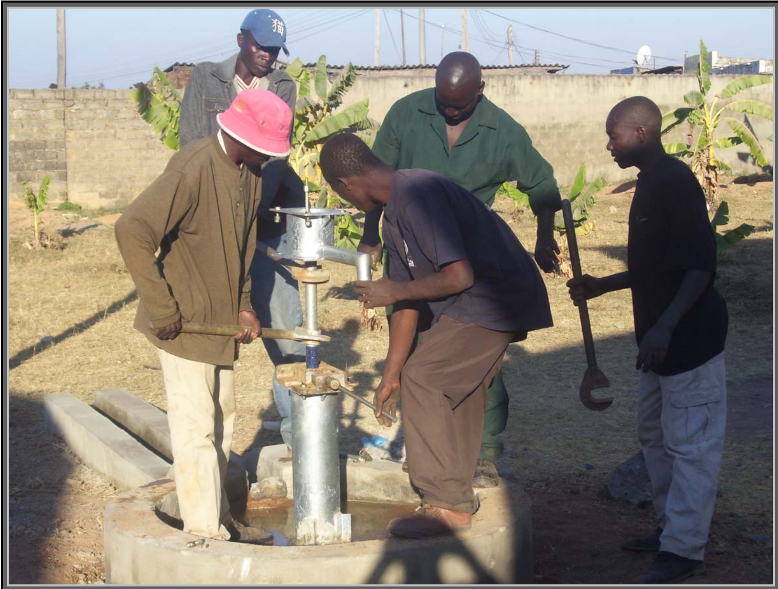
That's the new pump being fixed on the borehole.
