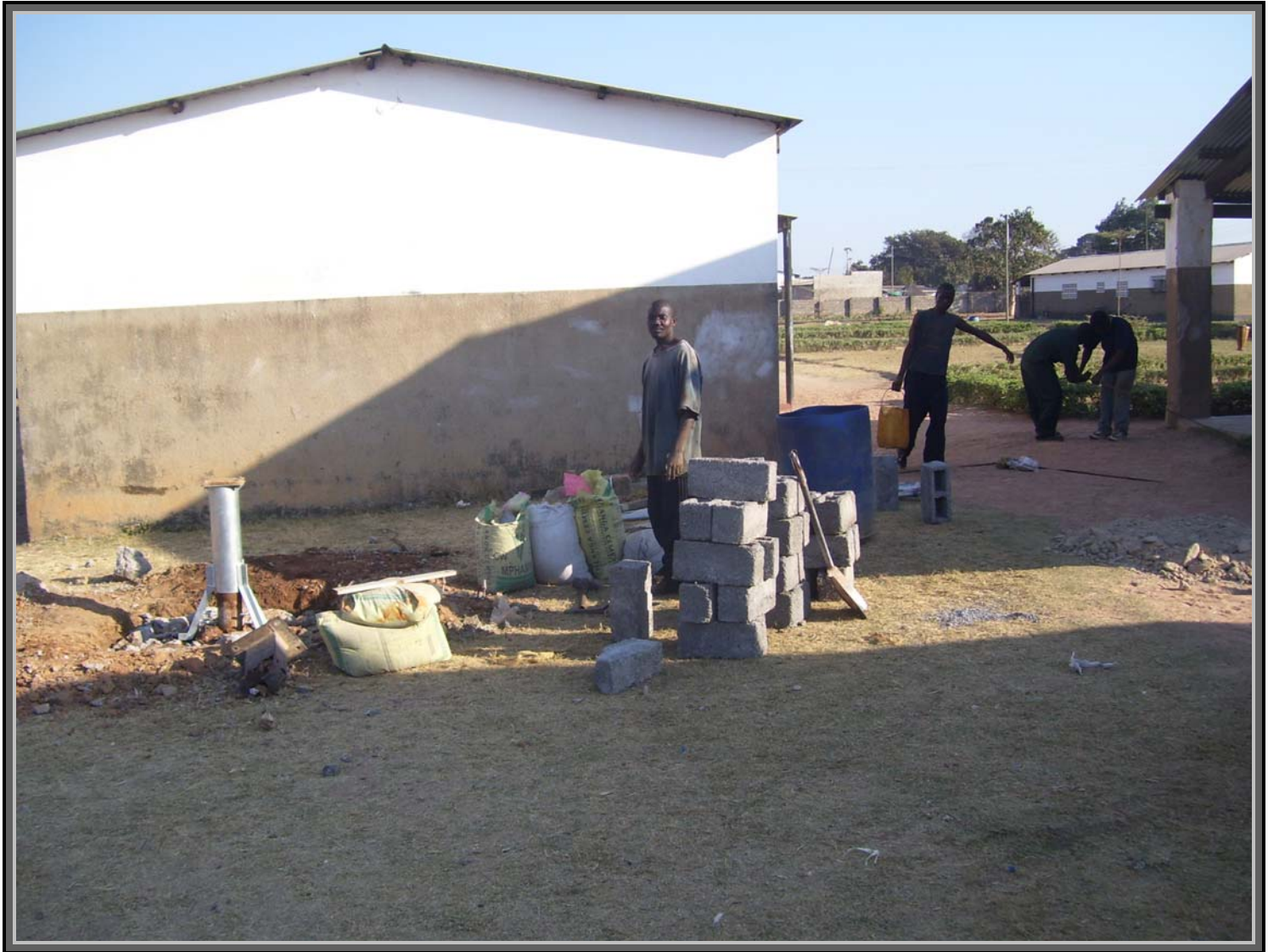
Apron construction, Nkwazi middle basic school.
